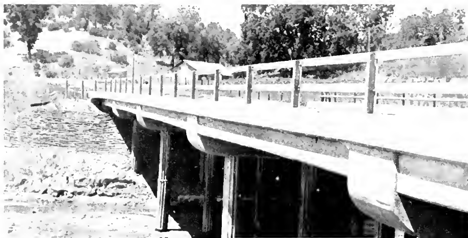
This is another view of Poso Creek Bridge railing
